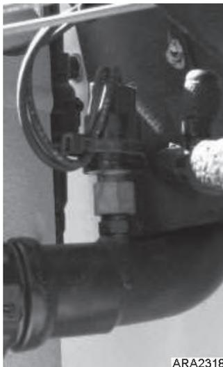
Figure 133: Low Pressure Cutout Switch Installed
