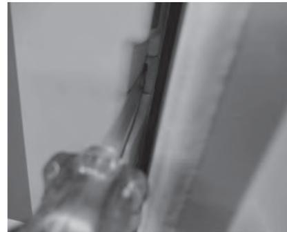
2. Move the screwdriver handle to the left to release the door catch from the box latch.
